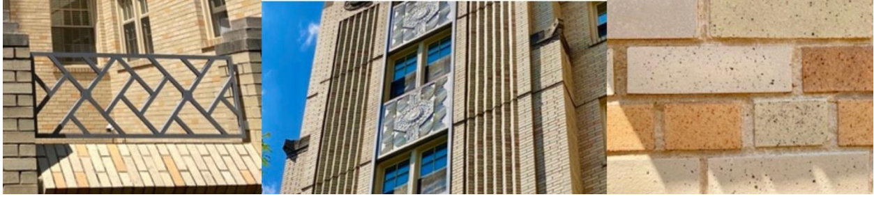
Fig. 29. Views of South Wing details: railings, bricks, and aluminum spandrels.
