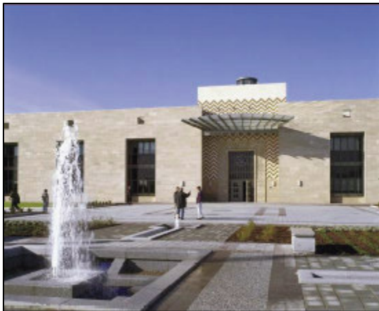
Tunis, Tunisia, NEC. Architect: Tai Soo Kim Partners Photo: OBO
