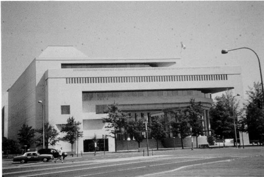
Figure 10 Arthur Erickson, Canadian Embassy, 501 Pennsylvania Avenue, N.W., Washington, D.C., 1978–89, Pennsylvania Avenue façade
