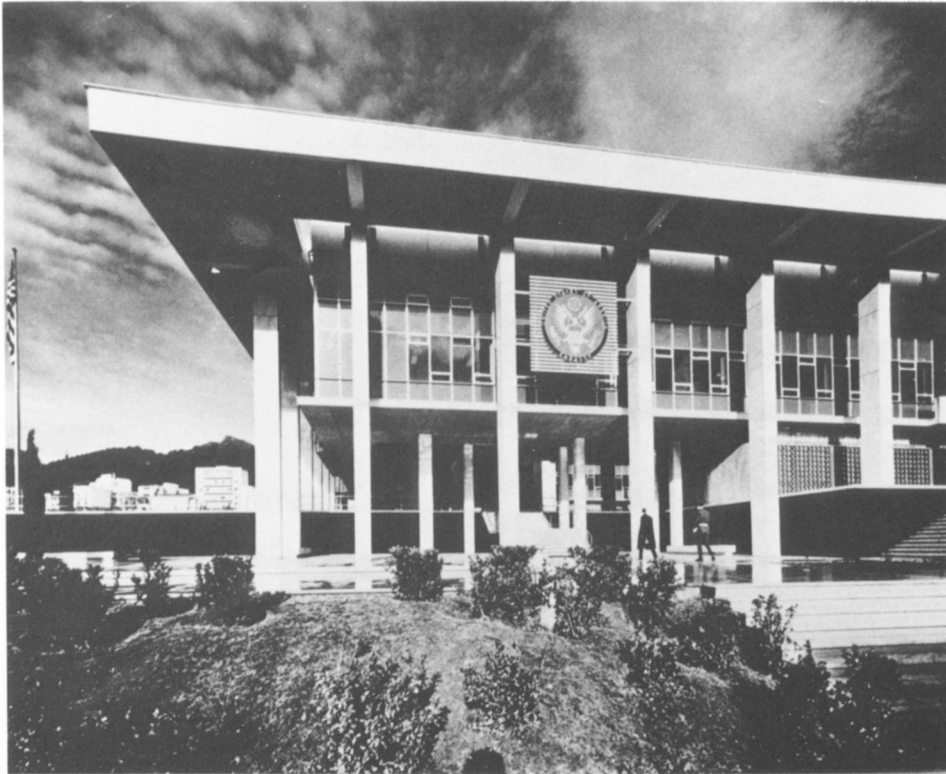
Fig. 8. Walter Gropius, The Architects Collaborative, U.S. Embassy, Athens, Greece, 1956–1961. See perforated tile screens at lower right (Department of State).
