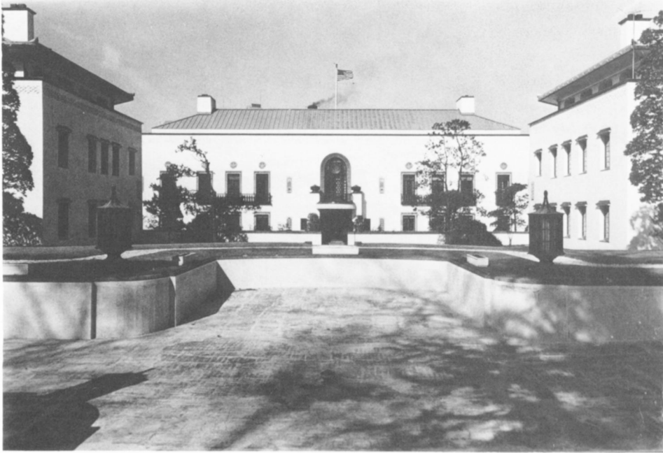
Fig. 2. Antonin Raymond and H. Van Buren Magonigle, U. S. Embassy Complex, office and residence, Tokyo, Japan, 1931, now serving as the ambassador's residence. Interior courtyard view across fountain. A new office tower, designed by Cesar Pelli and Gruen Associates, was completed in 1976 (Department of State).
