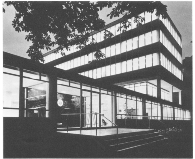
Fig. 4. Gordon Bunshaft for Skidmore, Owings & Merrill, U.S. Consulate, Frankfurt, Federal Republic of Germany, 1952 (Department of State).
