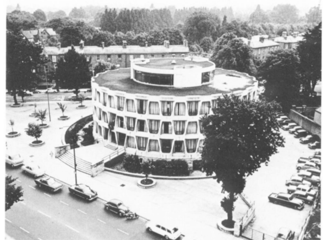
Fig. 23. John Johansen, U.S. Embassy, Dublin, Ireland, 1959–1964. Aerial view showing entrance with moat (Department of State/Pat Mohaghan, Fotoprint).
