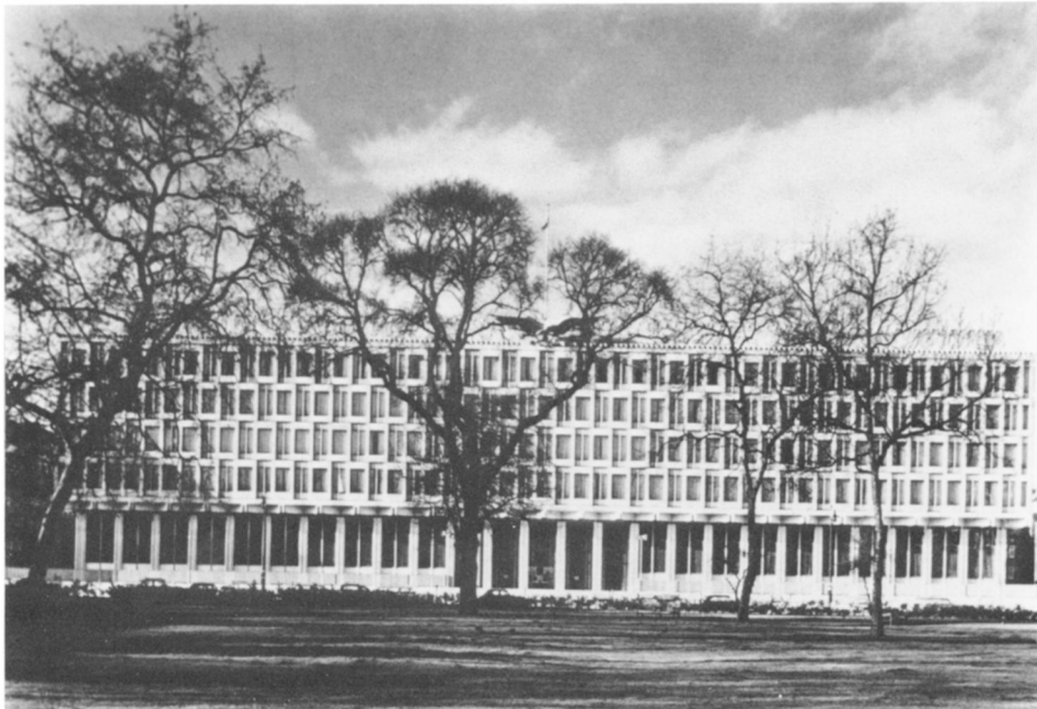
Fig. 25. Eero Saarinen, U.S. Embassy, London, England, 1956–1960. Façade from Grosvenor Square in 1963. Saarinen won the FBO design competition with a slightly different version of this building, which lacked the eagle over the entrance (Department of State/Balthazar Korab).
