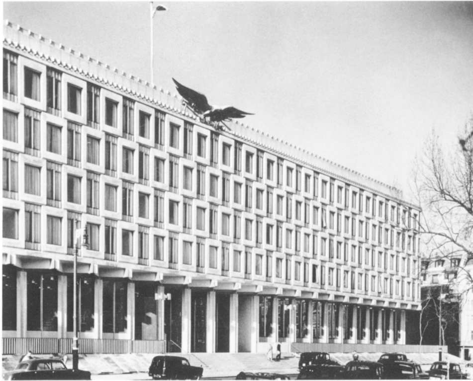
Fig. 26. Saarinen, London Embassy. Detail with eagle, raised base, wall articulation, and cornice decoration, seen from Grosvenor Square. Sash is operable. Cornice trim, window sash, railings, and the eagle are of straw-colored anodized aluminum (Balthazar Korab).
